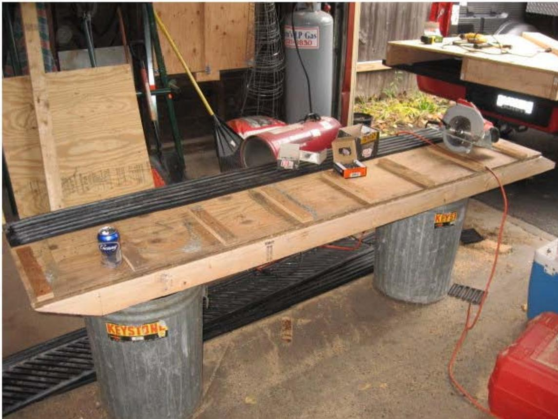
I built the 2x6 deck in the back of the truck. Here i am putting the blocking in the far end of the deck between the 3 joists. After, I spun it around and attached to the bed.
